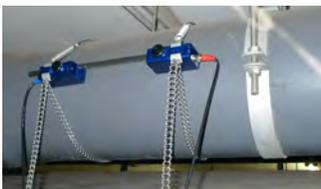
Since the ultrasonic transducer does not come into contact with the fluid, the measurement is:
